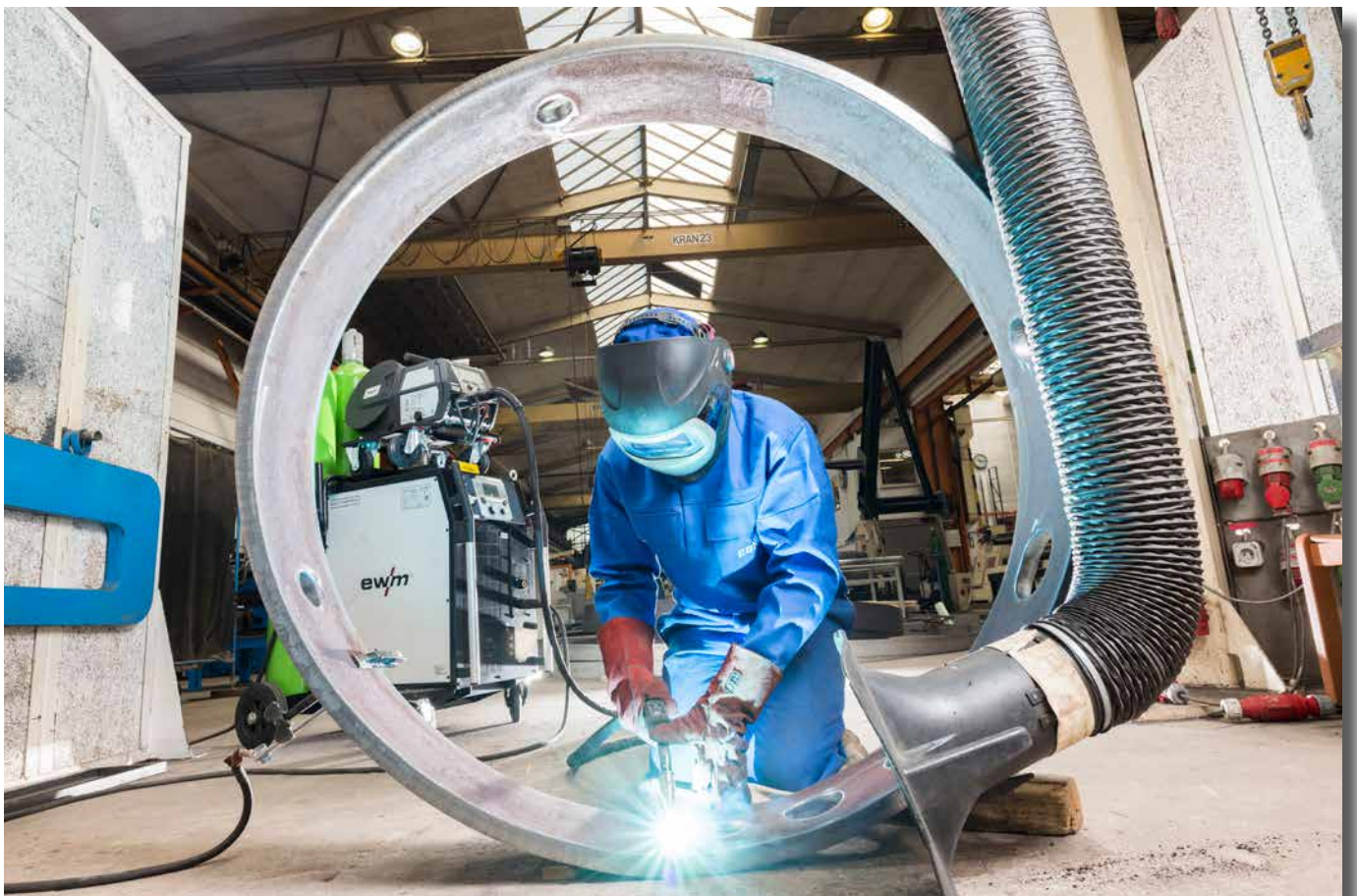
Welding a double V-butt weld on a steel ring using forceArc
